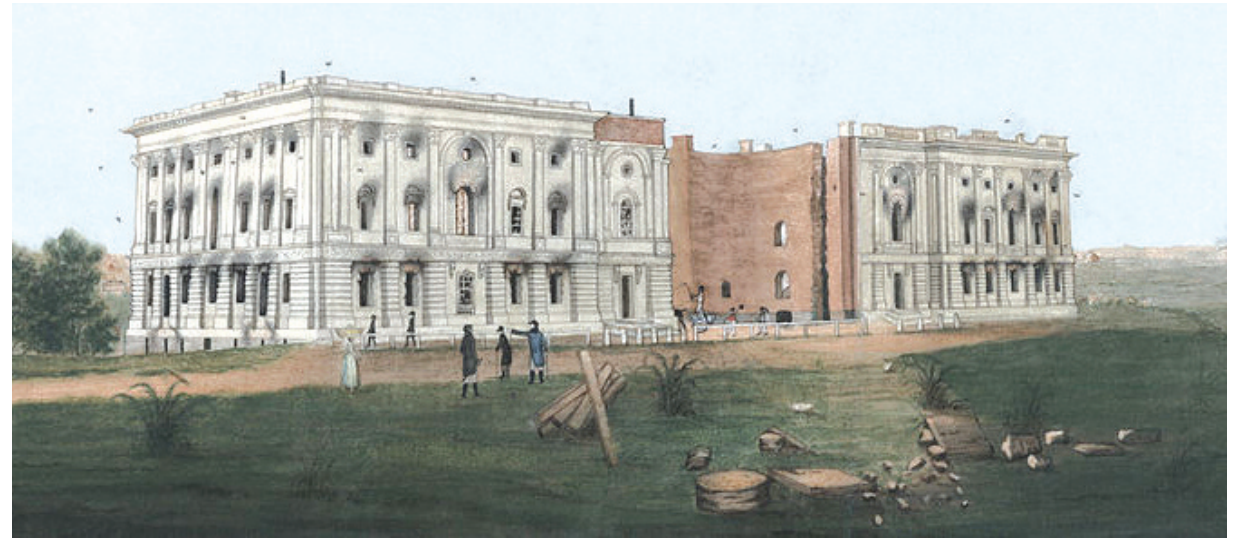
This drawing shows the ruins of the U.S. Capitol following British attempts to burn the building during the War of 1812. Depicted are fire damage to the Senate and House wings, damaged colonnade in the House of Representatives shored up with firewood to prevent its collapse, and the shell of the rotunda with the facade and roof missing. Historical drawing by George Munger.
